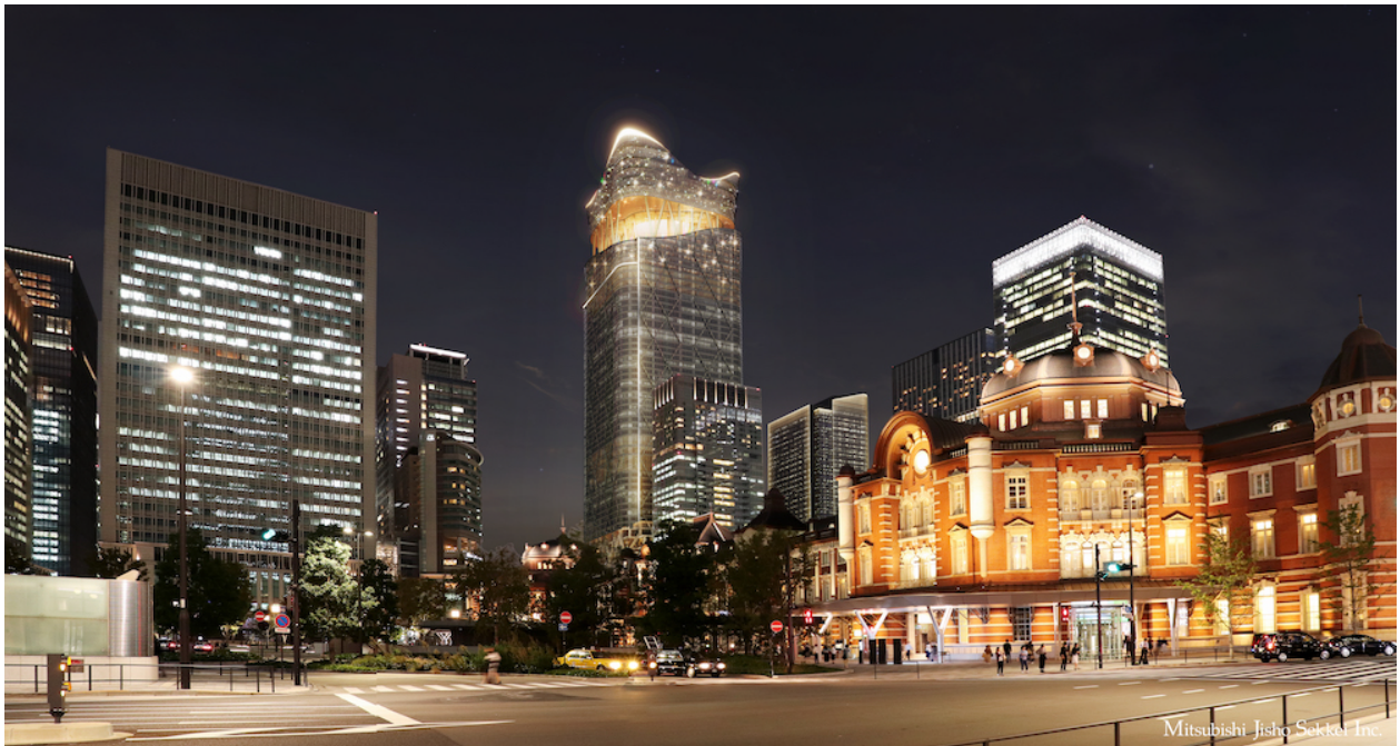
TOKYO TORCH viewed from west side of JR Tokyo Station (night view)
