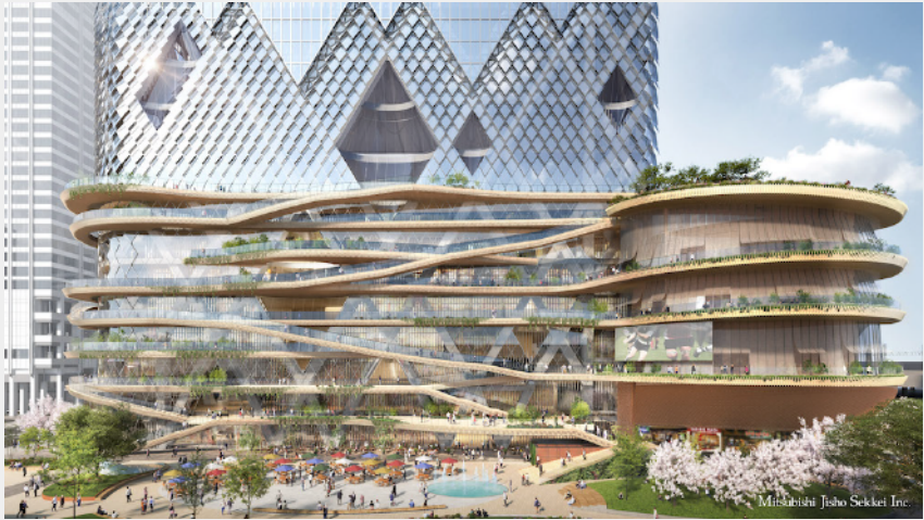
Torch Tower, Open-air walkway
