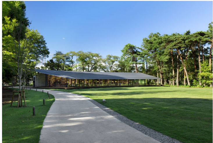
Photo: Nacasa & Partners Inc.
